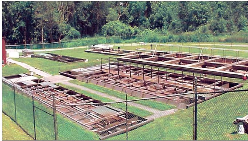
**Top photo: The 200,000 gpd Wimmerton Sewage Treatment Plant has a present flow of 160,000 gpd. Flow monitoring indicates severe infiltration in the collection system. Lower photo: Technician John Rosko watches the service truck monitor as Robert Paul feeds the camera into a lateral.**
