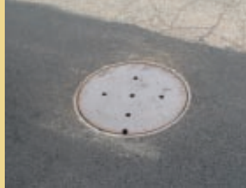
6 With MP Installed
